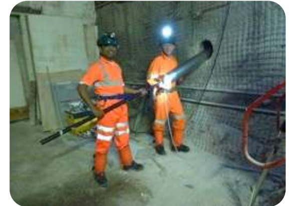
Bore hole detector installation
