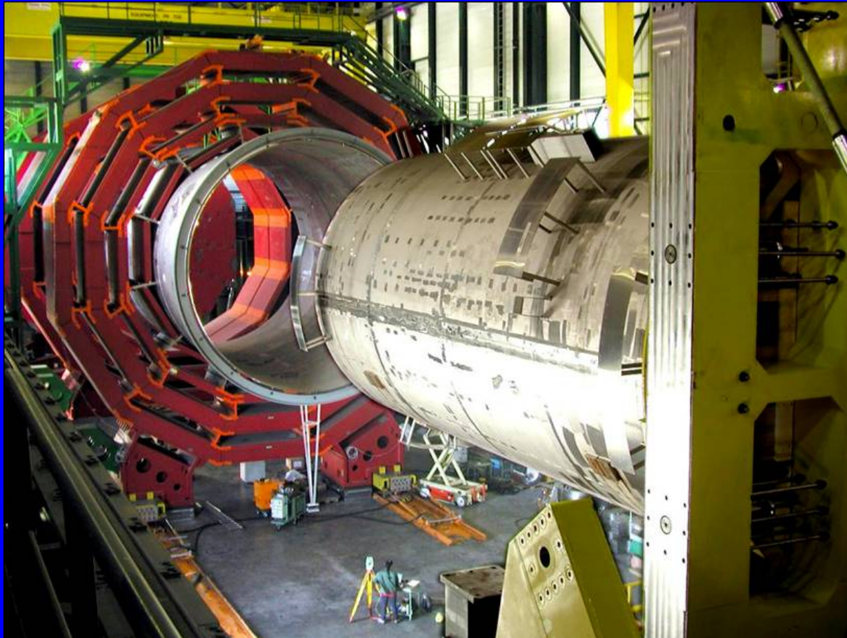
CMS: Inner Vacuum Tank insertion
